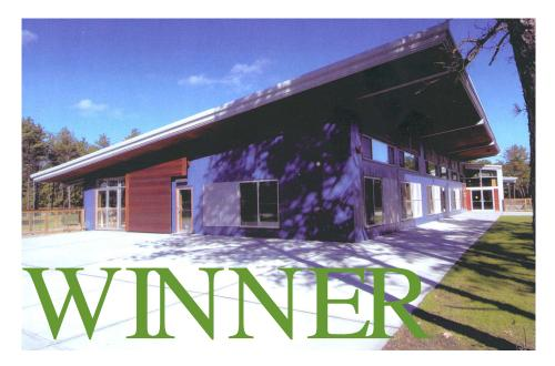
About the products: At the heart of the buildings construction is a 180' x 69' single - sloping clear span framing system with a 2:12 roof slope. It features concealed gutters, hidden fasteners, alternating pitches and a roof system that wraps down to become the walls in some areas. Kirby Building Systems manufactured the framing and roofing while Jenisys produced the metal wall panels.
